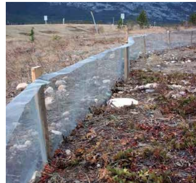
Figura 70: Barrera provisional para anfibios y reptiles. Fuente: Federal Highway Administration - U.S. Department of Transportation, 2011.
